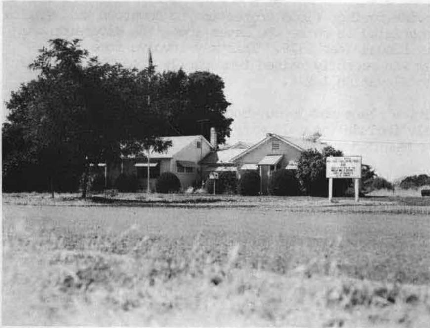
Caretaker's (damtender's) residence and headquarters. These buildings are part of the Mill Creek project.
